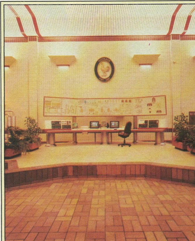
The brew hall in Courage's Bristol brewery shows the application of modern lighting techniques to a specialist environment. The hall houses an advanced computer console with four VDU screens which demand reflection and glare-free lighting. For this reason an uplighting system using wall and column-mounted uplights with asymmetric reflectors was chosen; lamps are 440W de luxe high pressure sodium to give excellent colour rendering. Special effect lighting is provided by 500W tungsten halogen spotlights recessed into the sloping ceiling and these employ red filters to enhance the colour of the coppers.
