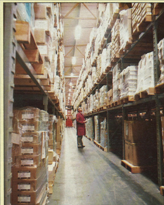
The stationery store at Barclays PLC, Milton Keynes, has ten narrow high racking aisles which were lit from 168 twin 85W, 1800mm trough reflector fittings mounted on the trunking, with a total installed load of 30.24kW. The illuminance at ground level was 100 lux. These were replaced with 104 Philips GTX luminaires each embodying one 58W, 1500mm fluorescent lamp. The specular reflector gives a narrow distribution of 2 \times 16^\circ so that an illuminance of over 100 lux is given at ground level, with good vertical illumination at all levels. The total installed load has been reduced to 7.28kW, a saving of 76%.
